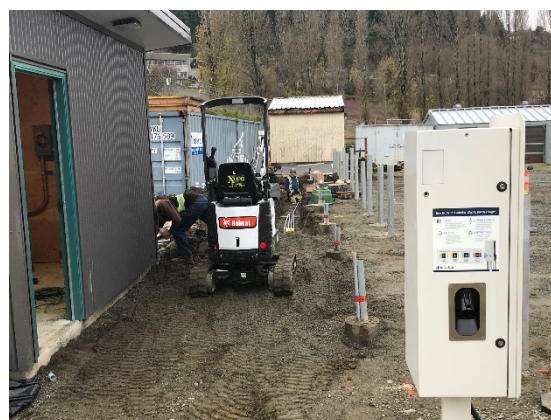
Figure 7. Installation of electrical infrastructure for the electric vehicle supply equipment (chargers) installed at School District 68
